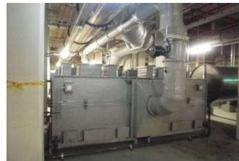
除臭常溫觸媒吸附塔 (Deodorization Catalyst Adsorber)
